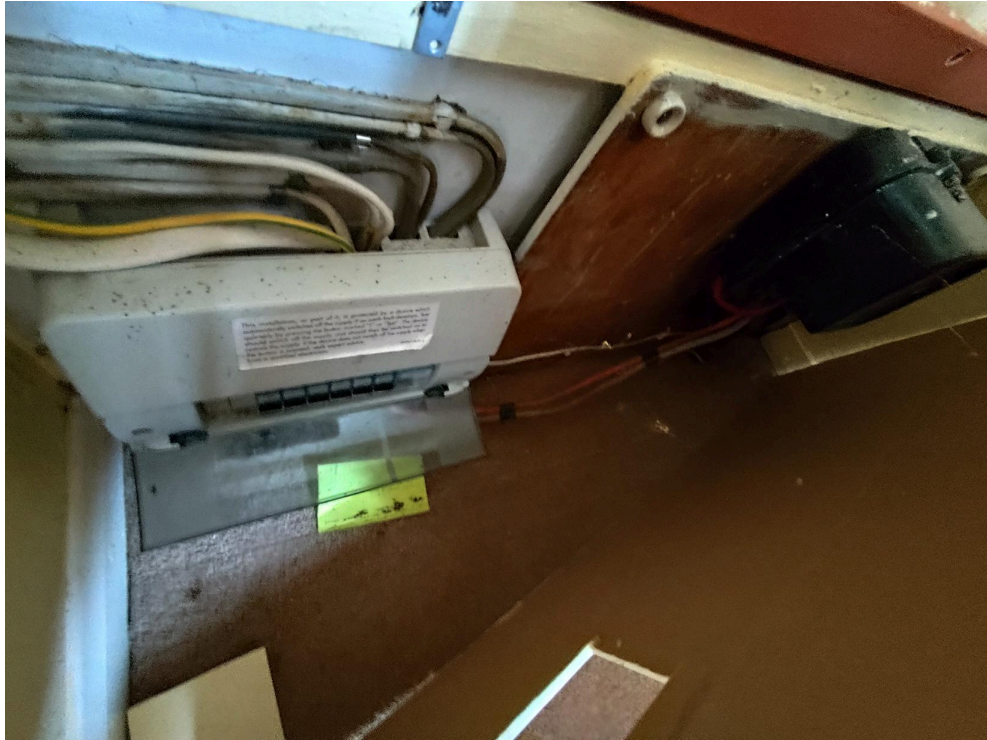
Electric Meter and Consumer Unit
