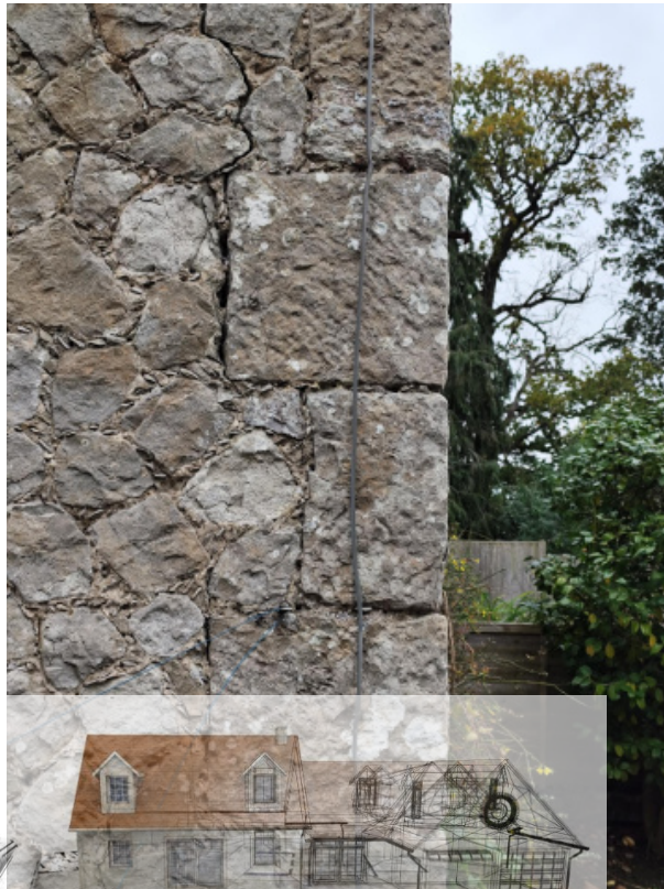
Crack to wall
