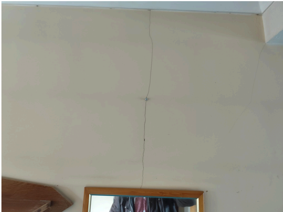
Hairline Wall Crack
