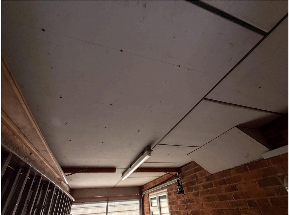
Asbestos sheeting in garage(2)
