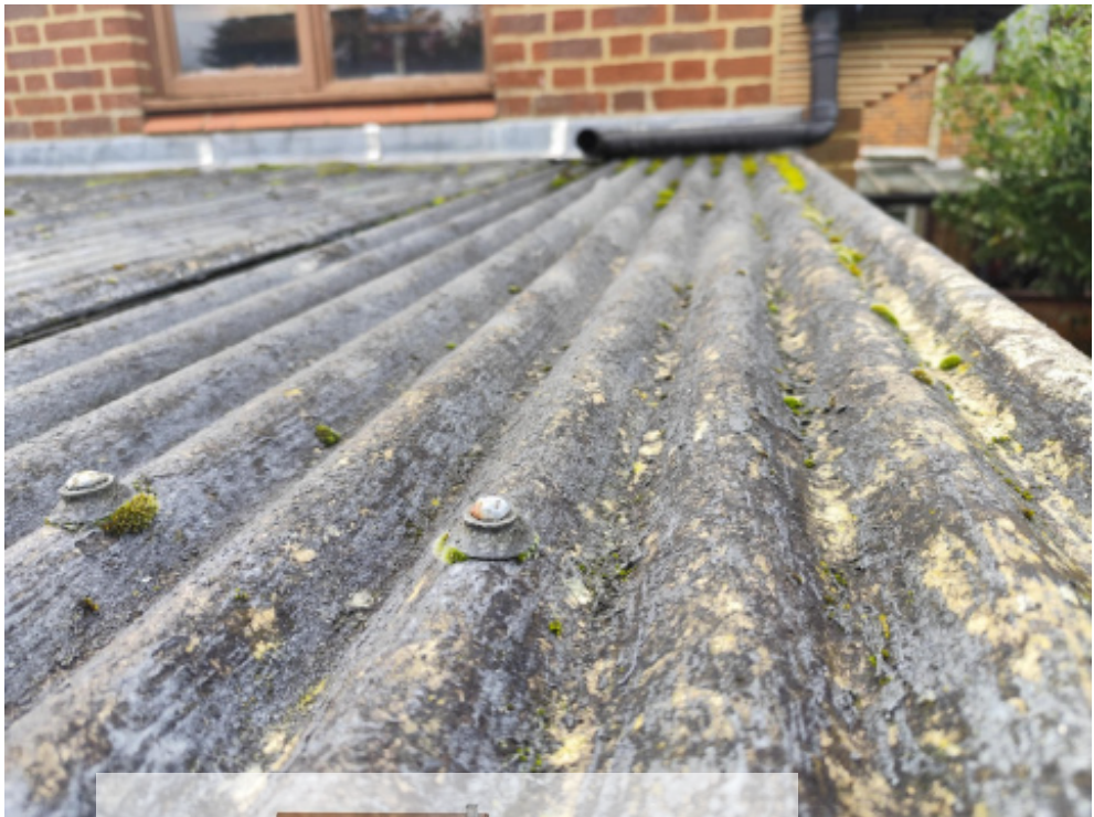
Corrugated roof containing asbestos material.
