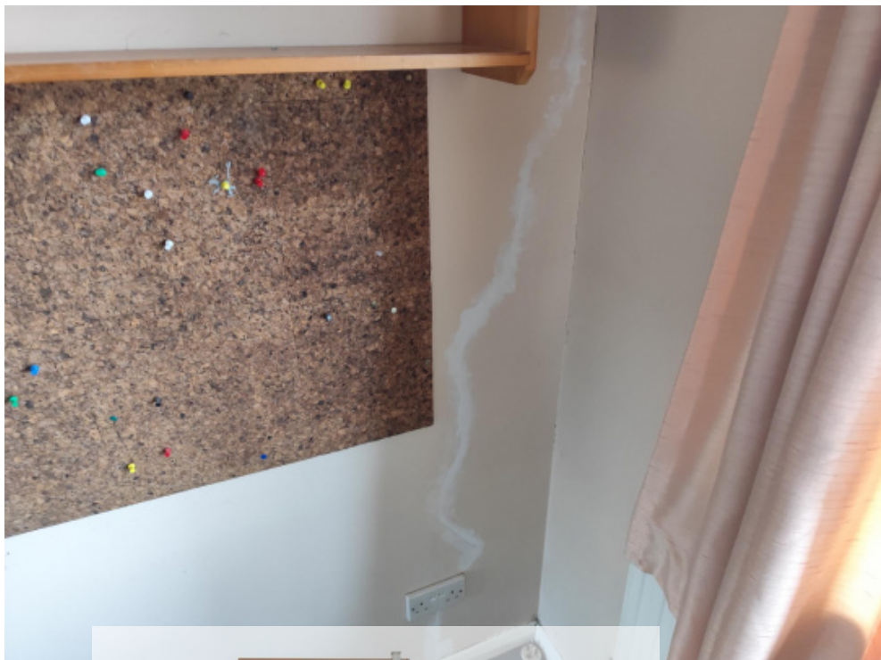
Repaired wall crack
