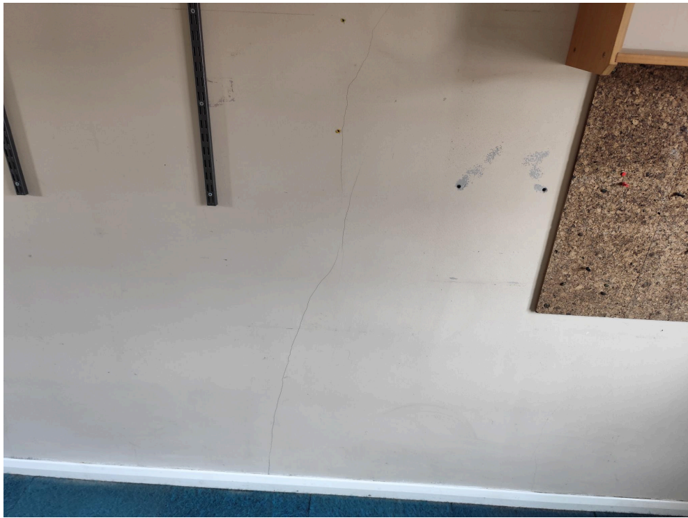
Hairline Wall Crack
