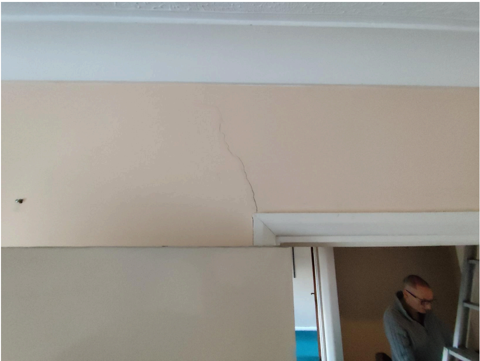
Hairline Wall Crack
