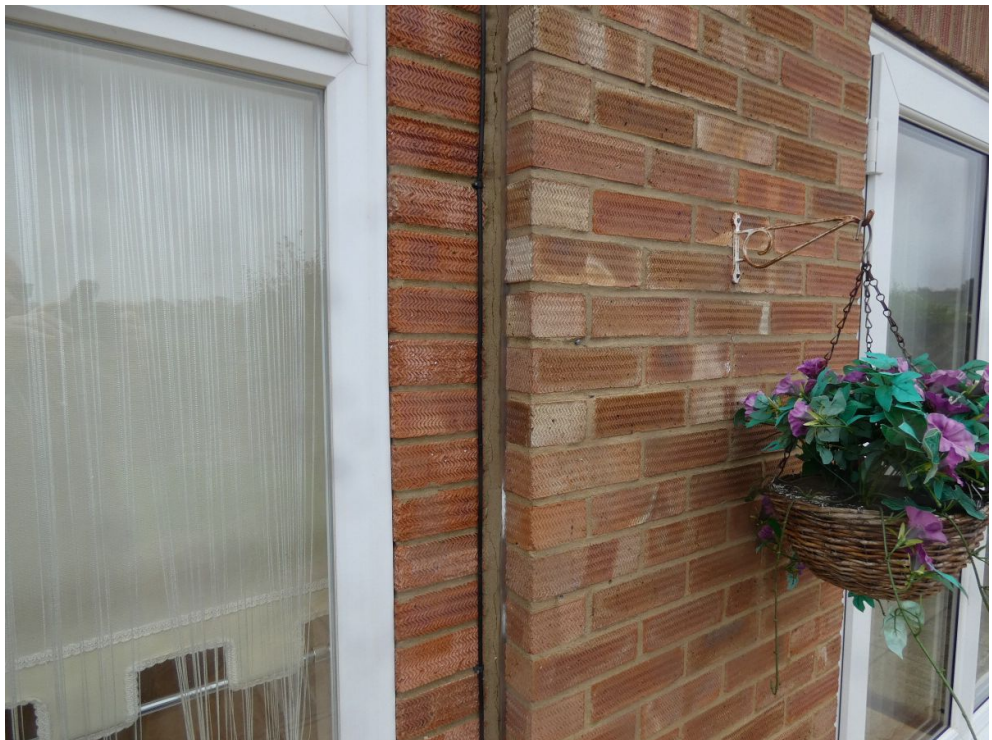
Crack between conservatory and rear extension
