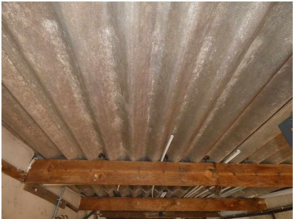
Asbestos sheet in garage
