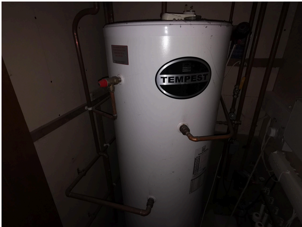
Unvented hot water cylinder
